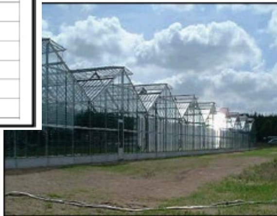
Fig. 3 A high-end closed bioreactor system. The worlds largest closed photo-bioreactor in Klötze, near Wolfsburg, Germany (Bioprodukte Prof. Steinberg; www.algomed.de ); the 700 m 3 are distributed in 500 km of tubes and produce up to 100 t algae biomass per year
